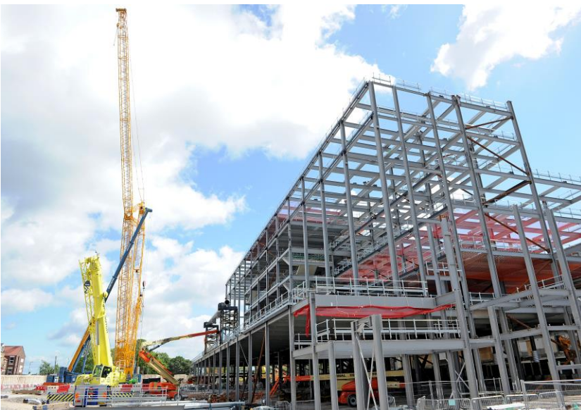
Image: Erecting the new steel structure at Anfield
